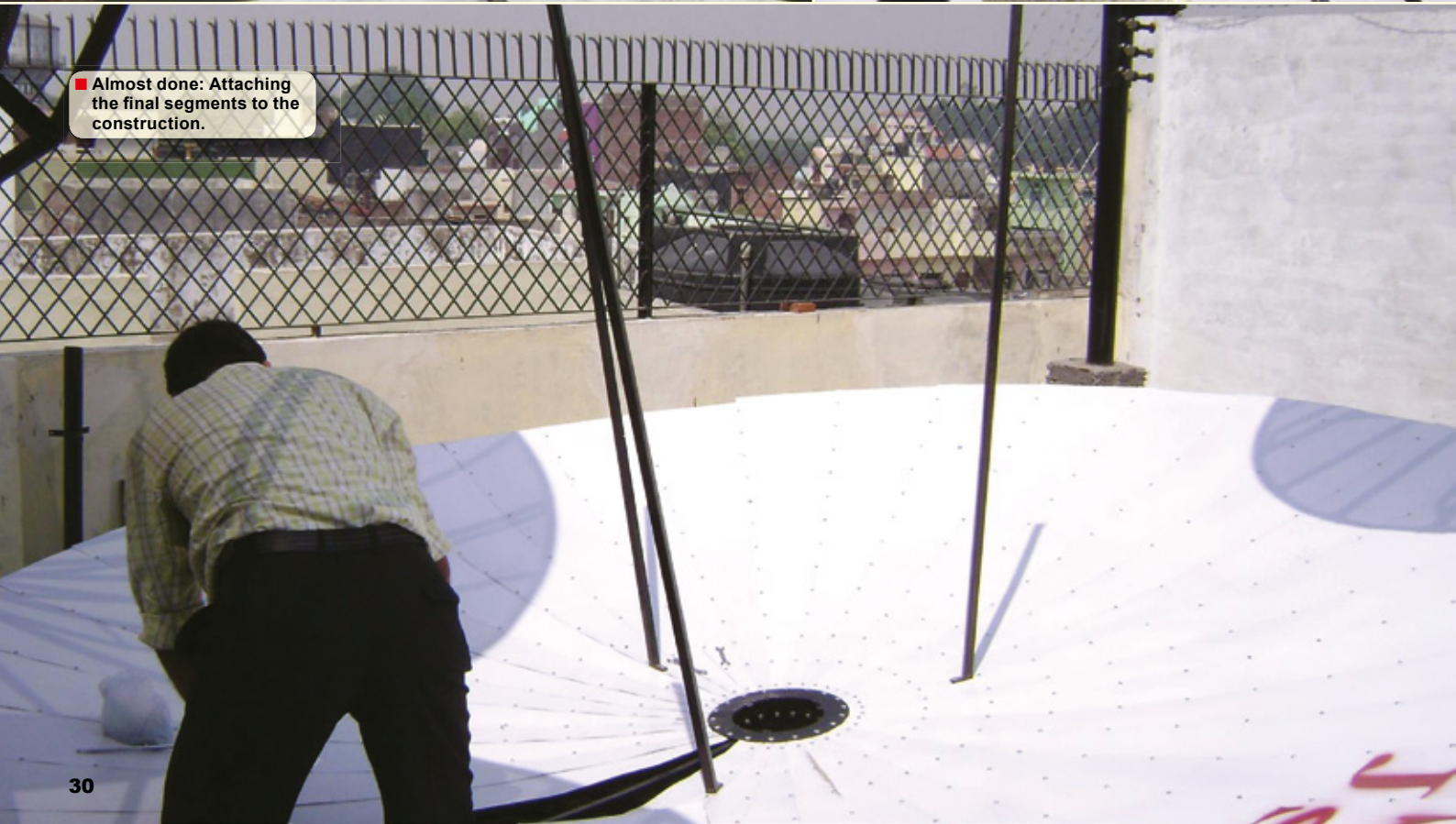
■ All support struts meet at the centre of the antenna.
