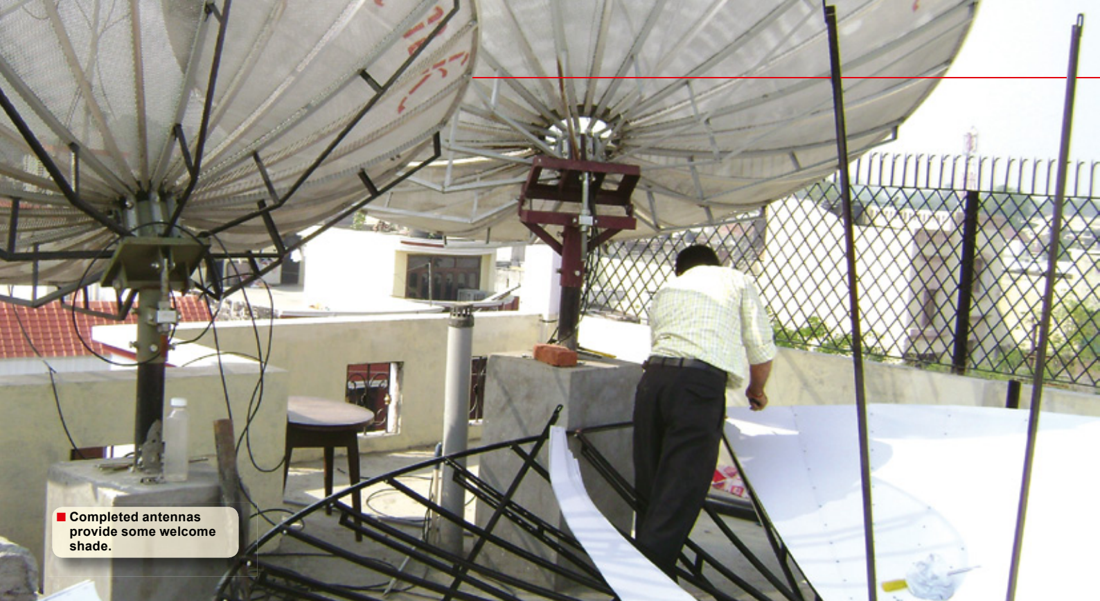
■ Screwing together the feed arms.
