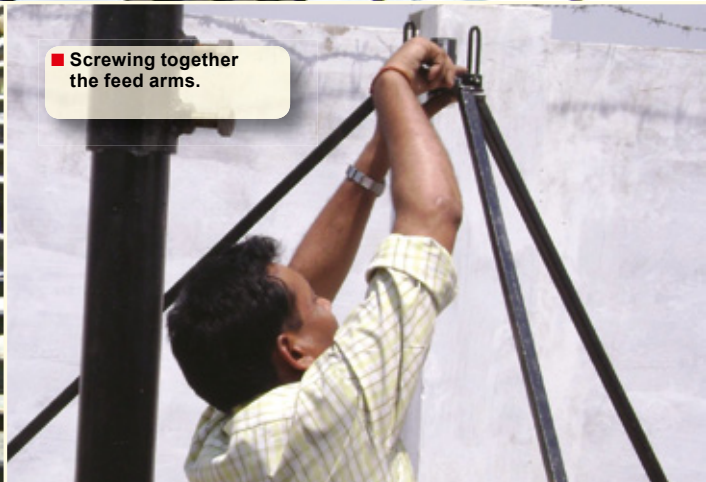
■ All support struts meet at the centre of the antenna.
