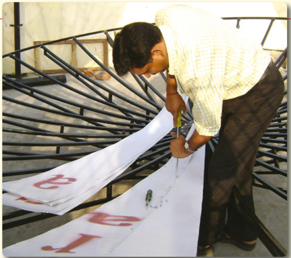
■ All individual segments are screwed onto the dish construction.
