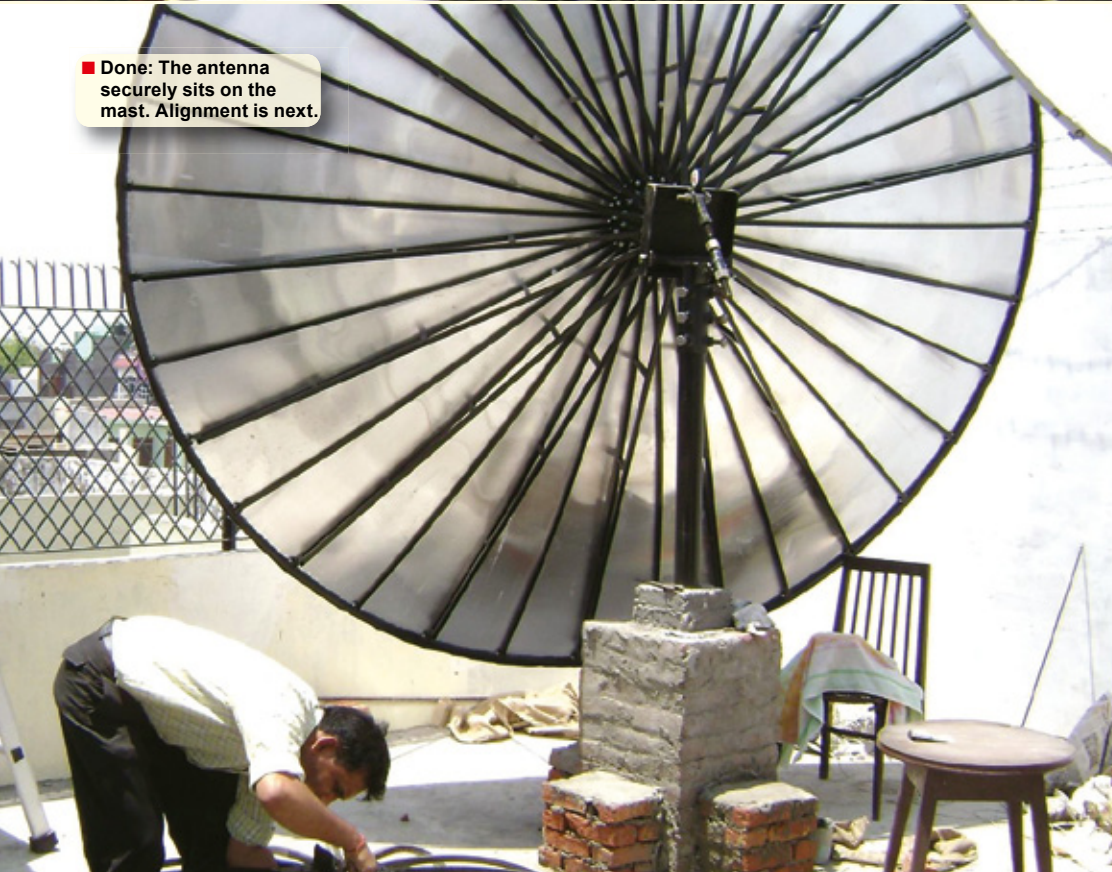
■ It took the helping hands of eight people to hoist the 2.4 m dish with its more than 200 kg onto the mast (visible in the front).
